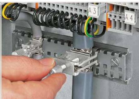
Tightening/removing a shield clamping saddle
