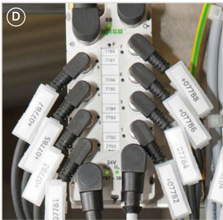
(C) Various versions of drag chain compatible, pre-assembled cables for power supply, system bus, fieldbus and separate pluggable connectors available as accessories! (D) Cable marking via marker sleeves in different lengths for various core diameters (211 Series)
