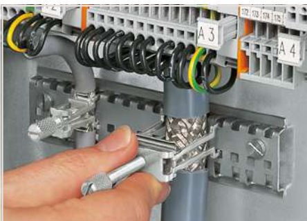
Fitting an additional clamping saddle
